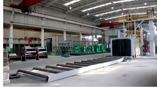
Ball Blasting and Paint
